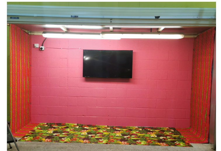
Installing In Rag Market
